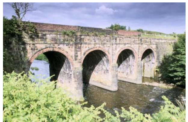
The Prestolee Aqueduct carries the canal over the River Irwell.
