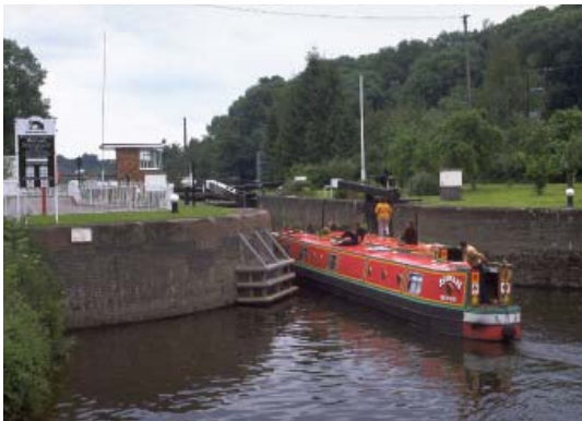
Holt Lock on the River Severn between Stourport and Worcester
