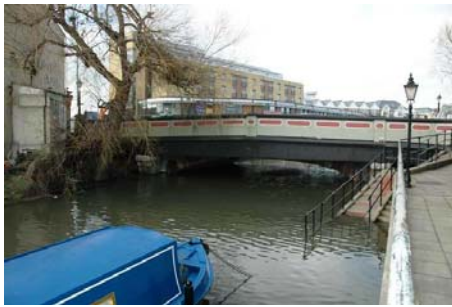
High tide in March 2006. The water came over the towpath and the boat couldn't get under the bridge.
