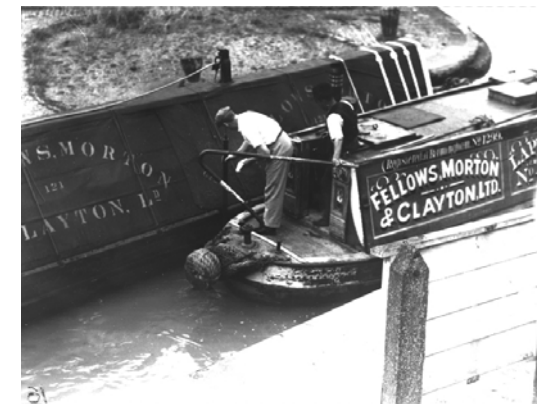
Here the toll clerk is gauging the load of a boat in the 1930s. He is holding the gauging rod against the side of a boat while the boatman watches.
