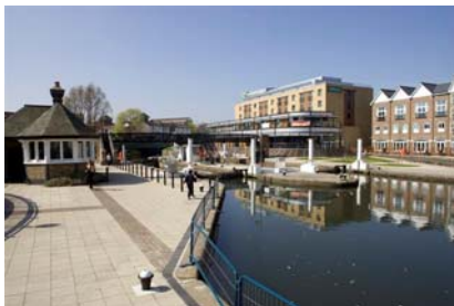
Brentford gauging locks today. Flats, offices and a hotel are to the right and the old Toll House is on the left.
