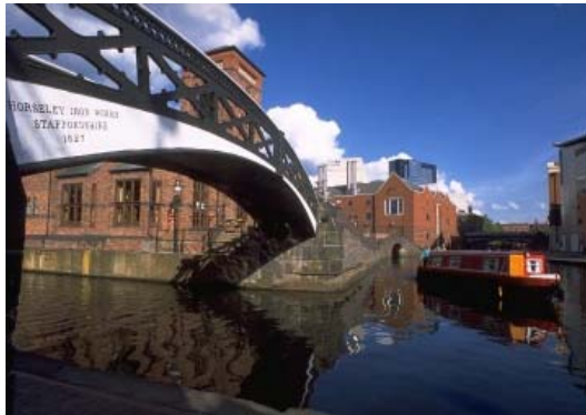
Thomas Telford straightened and shortened the Birmingham Canal in the 1820s.
