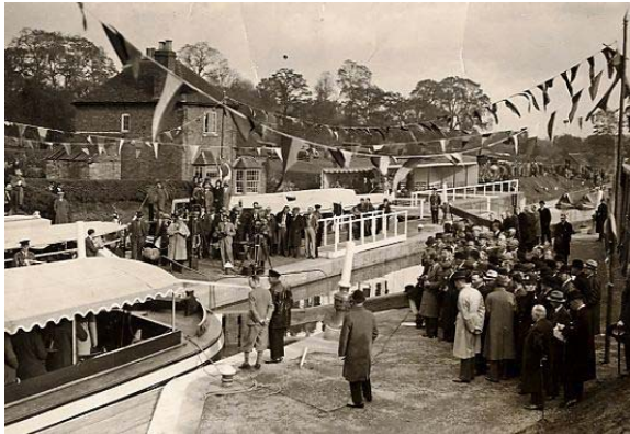
The Duke of Kent opened the new locks on 20 October 1934.
