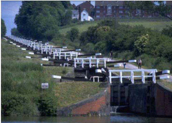
The flight of 16 locks at Caen Hill near Devizes was the last section of the canal to be completed in 1810
