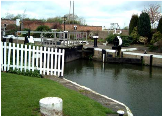
The gates at Torkey Lock
